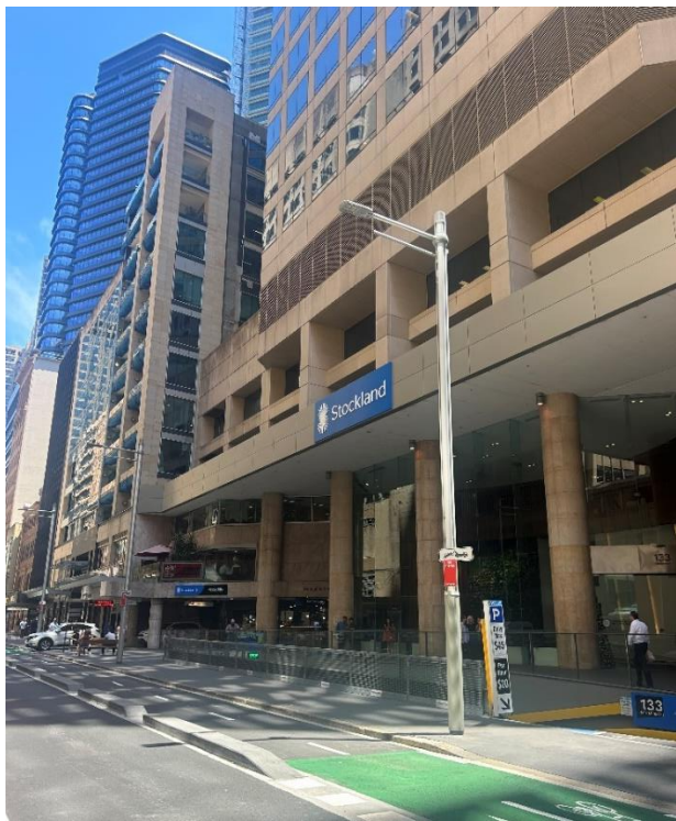
View of vehicular access ramp
